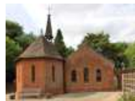
Sewards End with a 'fleche' comprising four-legged belfry and mini spire
