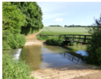
Thundridge Ford and footbridge over the Rib
